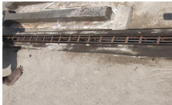
Fig 4. Casting of beams
