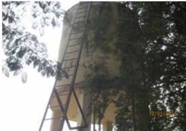
Fig.3.1 Image of the Water Tank
