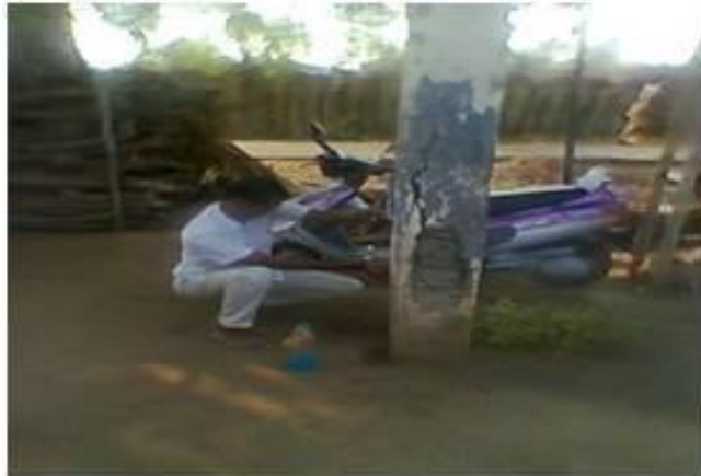
Fig.3.4 Half Cell Potential Difference Test being conducted on Column of the Water Tank
